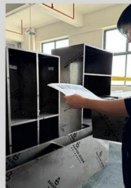
Pre installation inspection according to the drawings
